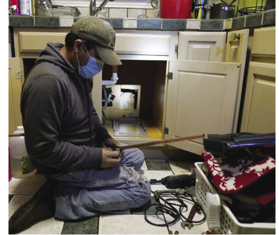
(TOP) Contractor Roberto Valerio works on repairing a broken pipe in the home of Nora Espinoza in Dallas. The pipe broke during freezing temperatures brought on by winter weather.
